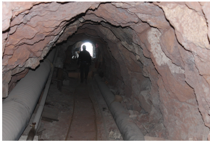
Figure 1. Dike tunnel in Tenerife Island (Western)
