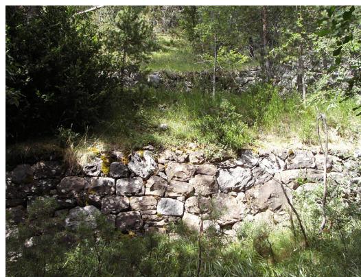
Figure 6. Actual state of masonry in the left bank
