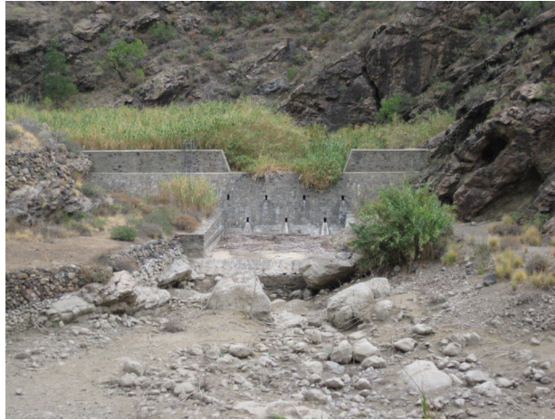
Figure 3. Dam of sediments in a ravine at Gran Canaria Island (Eastern)
