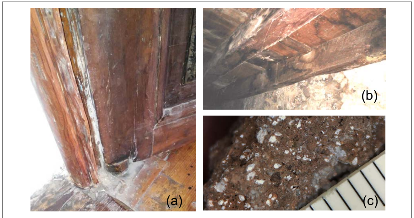
Fig. 2: Building elements selected for the study: (a) wooden doorpost, (b) wooden joist and (c) coating mortar, where the separation between the measurements of the ruler is 1 mm.
