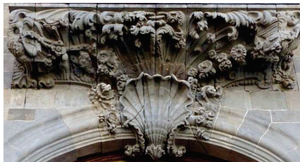
Fig. 2 Ornamentation applied to the main doorway of the church of "Nuestra Señora de la Concepción" (La Orotava)
