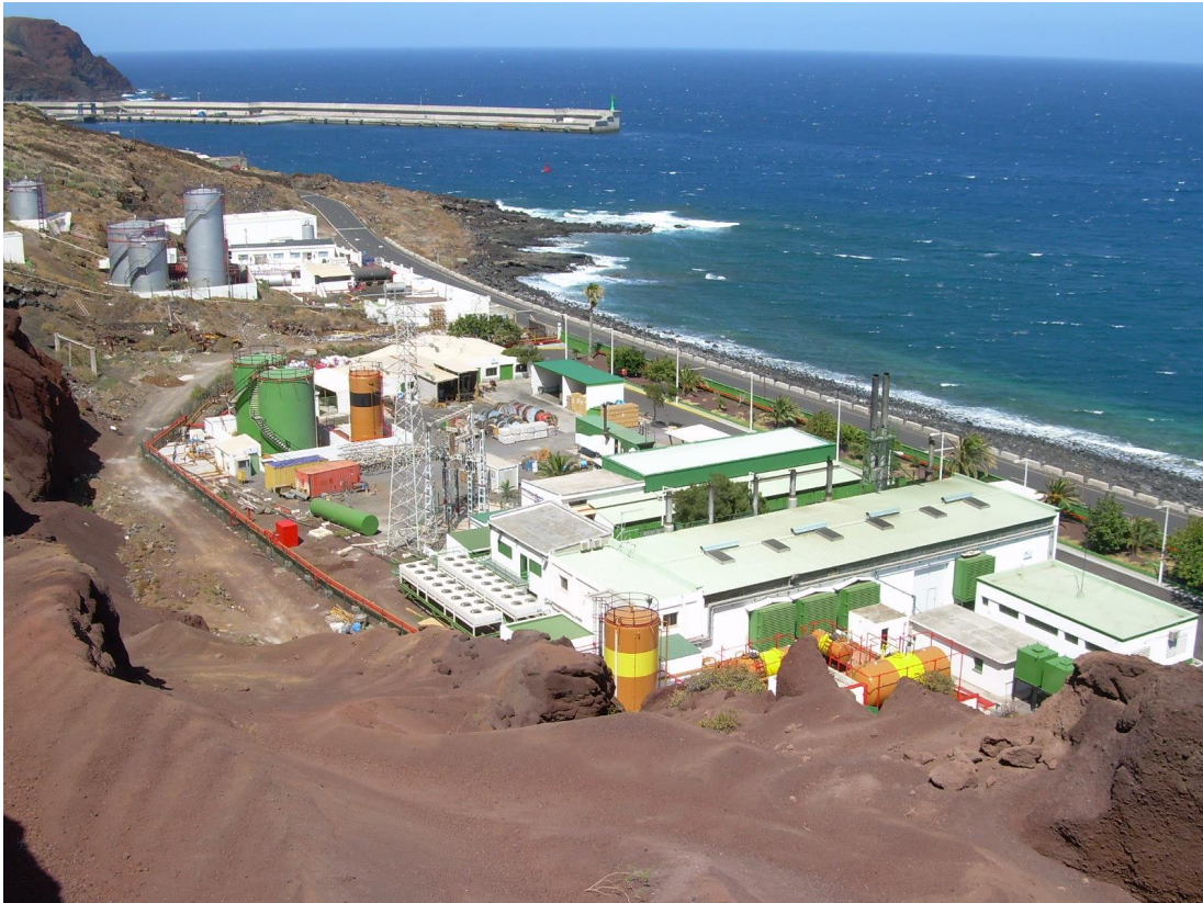
Figure 2. Diesel Electrical Power Plant on the island of El Hierro, Canary Islands
