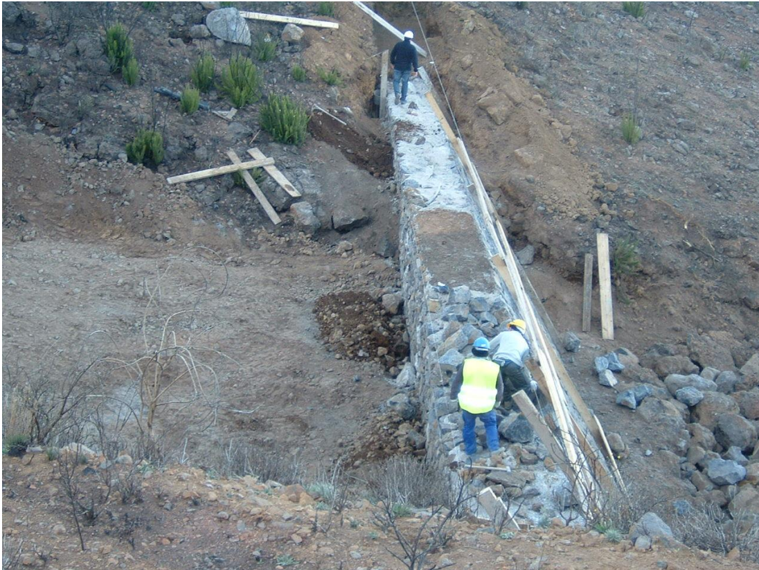
Figure 2. Construction of a sediment retention dam
