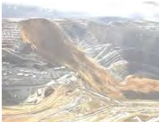
Figure 2.8. Landslides on slopes due to mining activity
