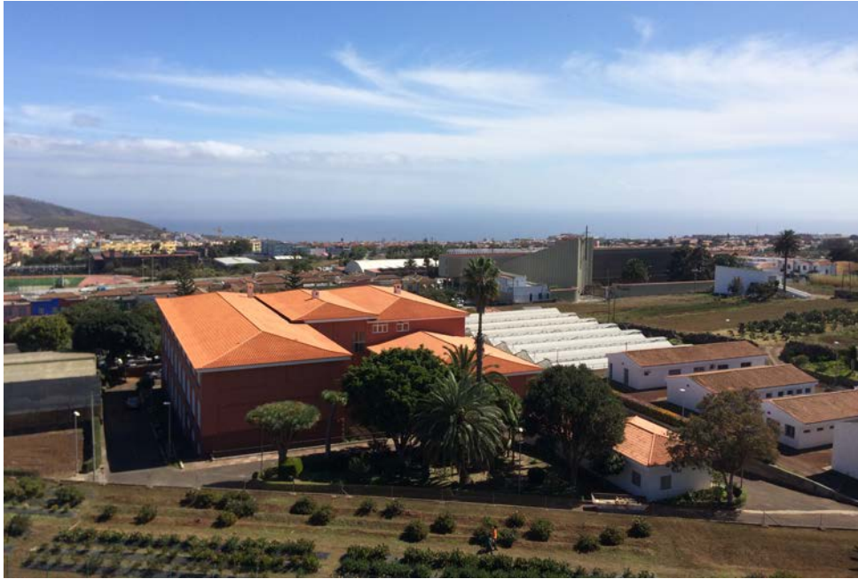
Figure 1. Facilities of the University of La Laguna School of Agricultural Engineering
